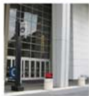
1. Building C entry
